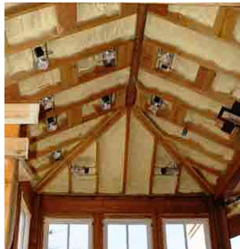
Foam insulation sprayed in attic
